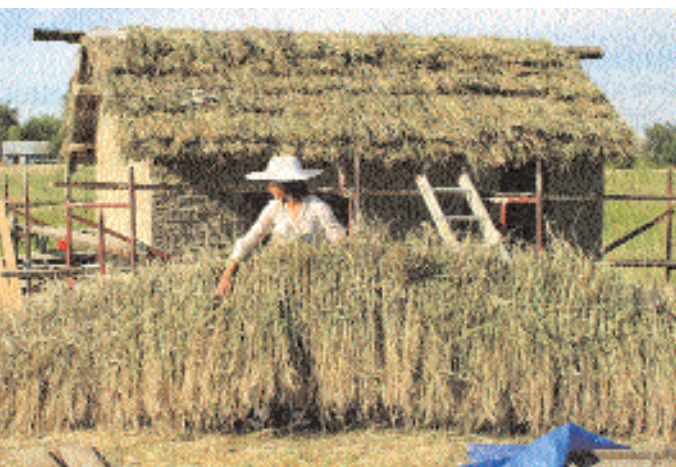
Native grasses are cut and bundled into approximately 60 cm (2 ft) square shingles for thatching the roof. They are layered using a wet clay and lime mortar over the lath. This long strip is about to be raised for the ridge.
