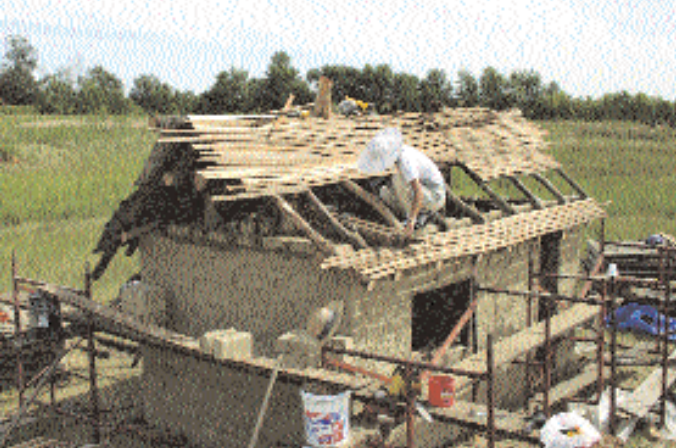
Salvaged lath from old barns is used to provide a base for applying the grass thatching roofing.
